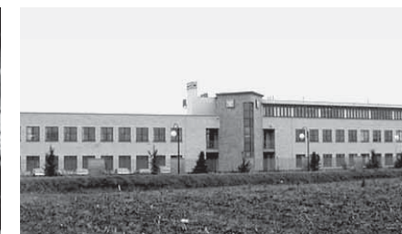
PAGAZZANO (BG) - SHOWER ENCLOSURES
